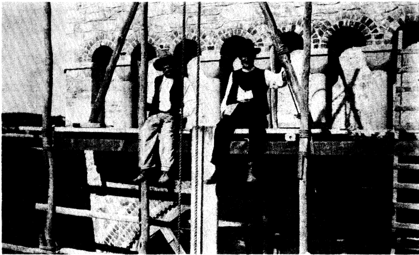
Geraldton Cathedral Stages of construction.
