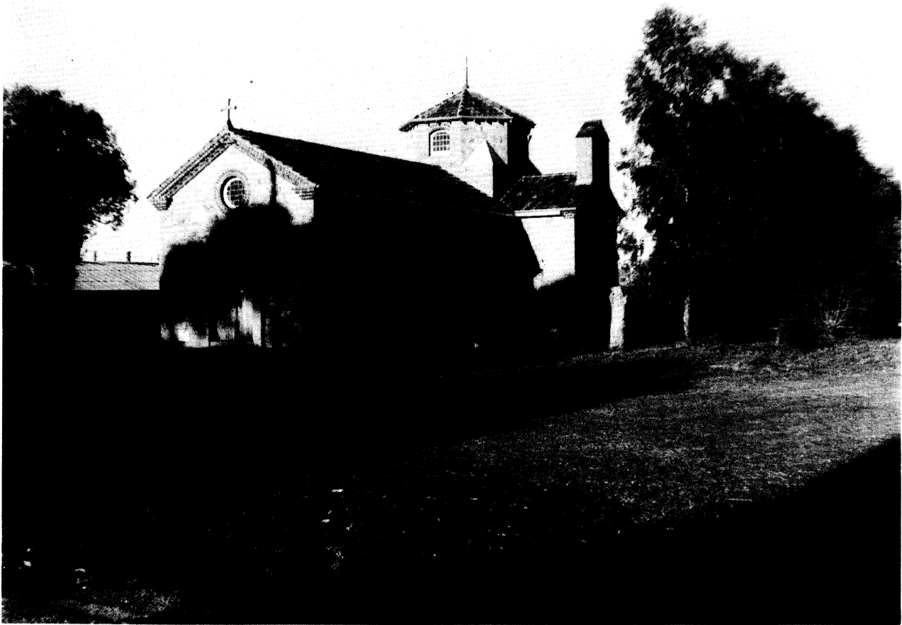
St Lawrence's, Bluff Point: the original church. The nave now completely removed. and a modern brick octagon attached to the transept.
